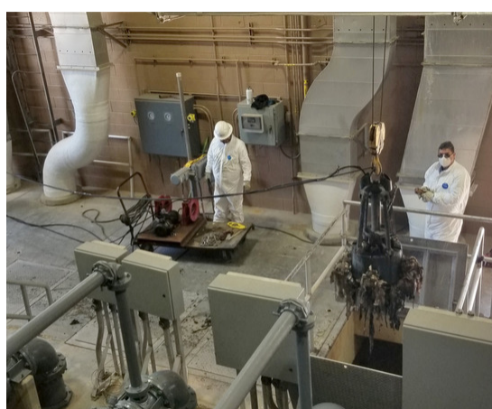
Wipes and rags are removed at the Haskell Wastewater Treatment Plant.
